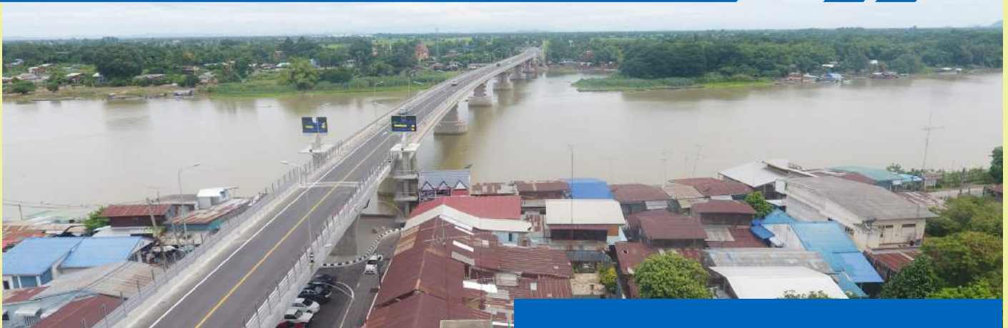
Chao Phraya River Crossing Bridge at Manorom District in Chai Nat Province Construction Project.
