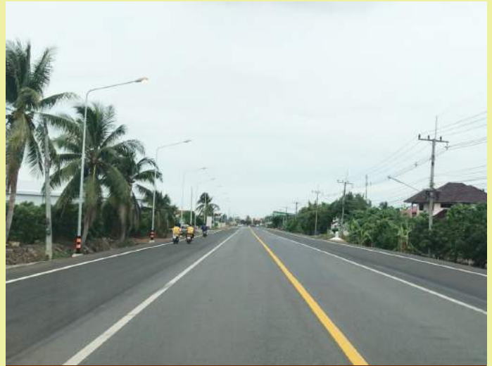
The Road Construction Project of Road CCO 3026 intersection. 331 - Ban Klong Rong Rouy, Plang Yao District, Chachoengsao Province
