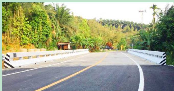
Maintenance Project as disaster on Road RNG 5036, Rural Road RNG 1004 intersection, Ban Klong Jan, Kra Buri District, Ranong Province
