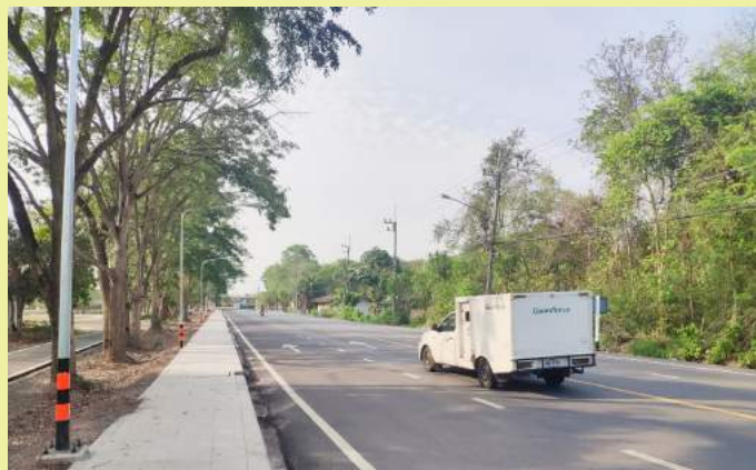
The Road Construction Project of road CCO 4023 intersection highway no3347 - Ban Khwai Khao Hak Ratchasat District, Bang Khla Chachoengsao Province.
