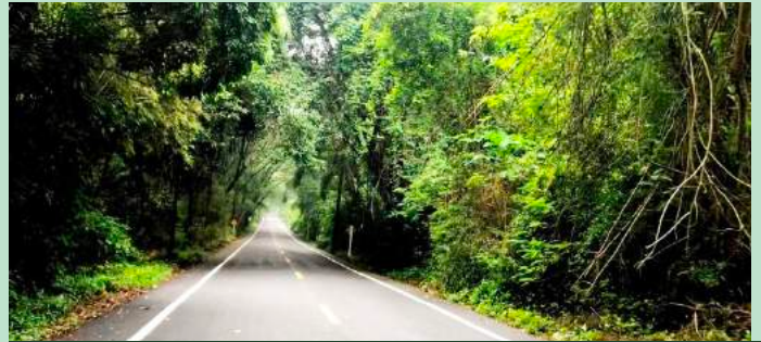
Maintenance Project on Road SRI 1003 intersection Highway No. 2 – Chet Khot Waterfall, Keng Koi District , Saraburi Province
