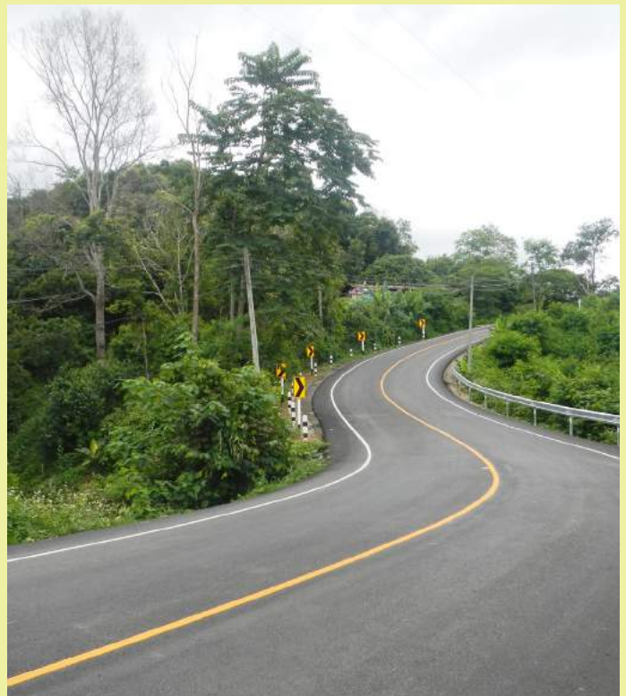
The Construction Road no.3037 intersection highway no.11 Ban Mai Mok Jam, Mae Suai District, Chiang Rai Province
