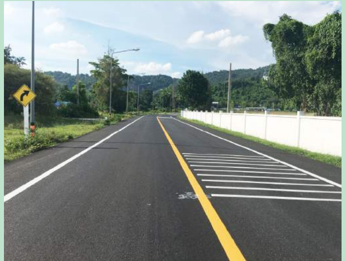
Maintenance Project for Para Asphaltic Concrete Road with Pavement In - Place Recycling Method on NYK 2013, Highway No.33 Intersection - Inpracharam Temple, Ban Na, Nakhon Nayok Province.
