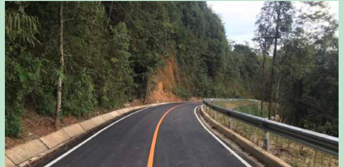
Maintenance Project as disaster on Rural Road CMI 4030 – intersection Highway No. 1096 to Huai Nam Dang National Park, Mae Taeng District, Chang Mai District
